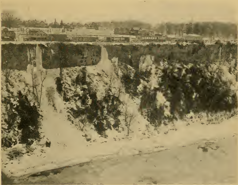
COMMERCIAL NIAGARA—THE CANADIAN BANK BELOW THE BRIDGE.
